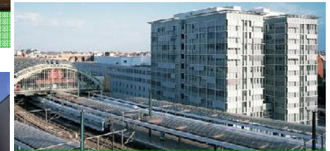
Railway station 1,250 kW
